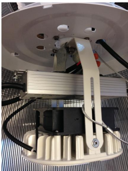
Typical 400W High Bay lights are an easy retrofit. The LED driver replaces the ballast in the ballast box. The Ultimate LED head is then screwed into the mogul base and the wires are connected.
